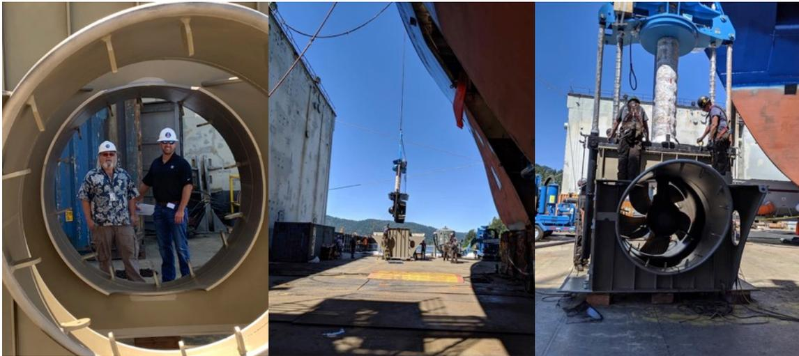
*Paul M. & Gaston ZF Marine Bow Thruster being installed in hull insert (photos Paul M.)*
