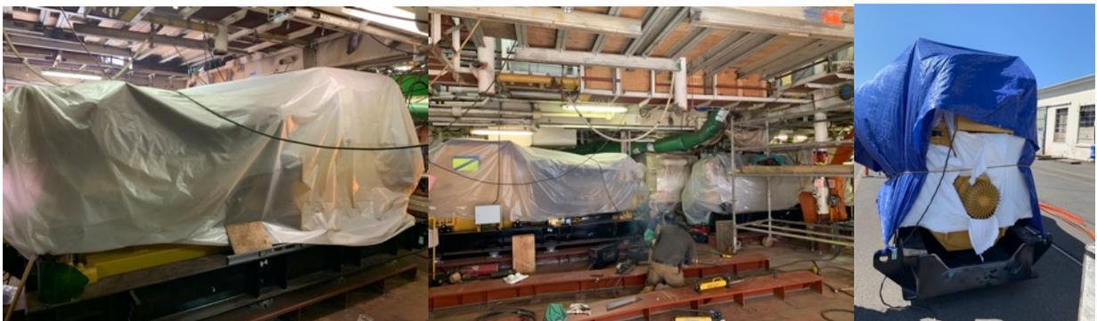
*C32 installed and foundation for first 3516 being welded in place; 3515 with modified skid*
