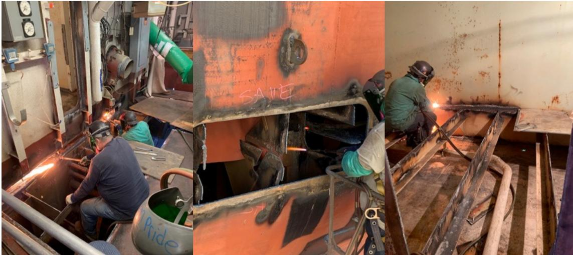
*Steel Work in forward Starboard area of engineroom & in potable water tank*
