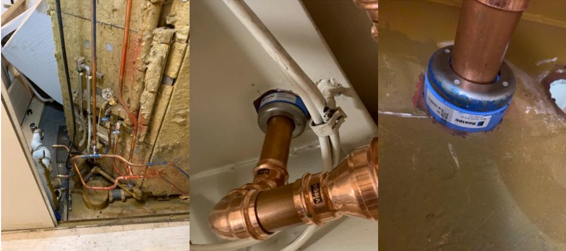
*Shower piping work; New Roxtec fittings for piping pass thru deck and bulkheads*
