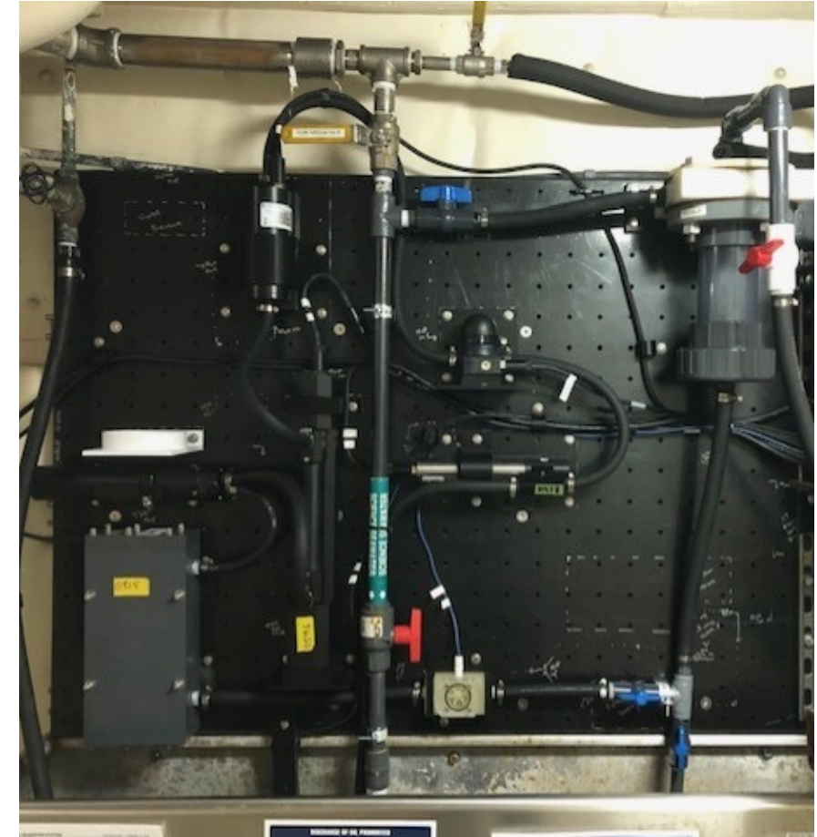
Port Side SSW Wall
