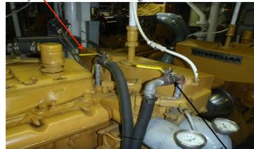
Generator jacket water from heat exchanger.
