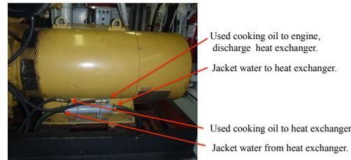
Figure 3. Cooking oil heat exchanger.
