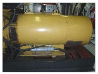
The generator was modified April of 2008. Approximately 300 gallons of used cooking oil have run through the generator's engine, providing ~4 days of power. The cooking oil was used only while the vessel was at the dock. The R/V CAPE HATTERAS found that the logistics and supply consistency were the biggest challenge of the operation.
