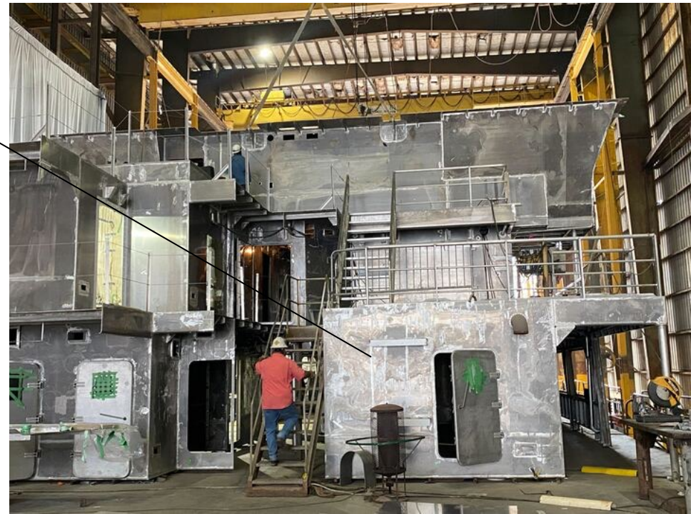
Aluminum superstructure, looking forward
