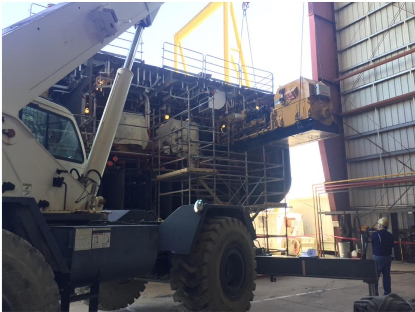
V1: Weighing Blue Drives before installation into Mod 32
