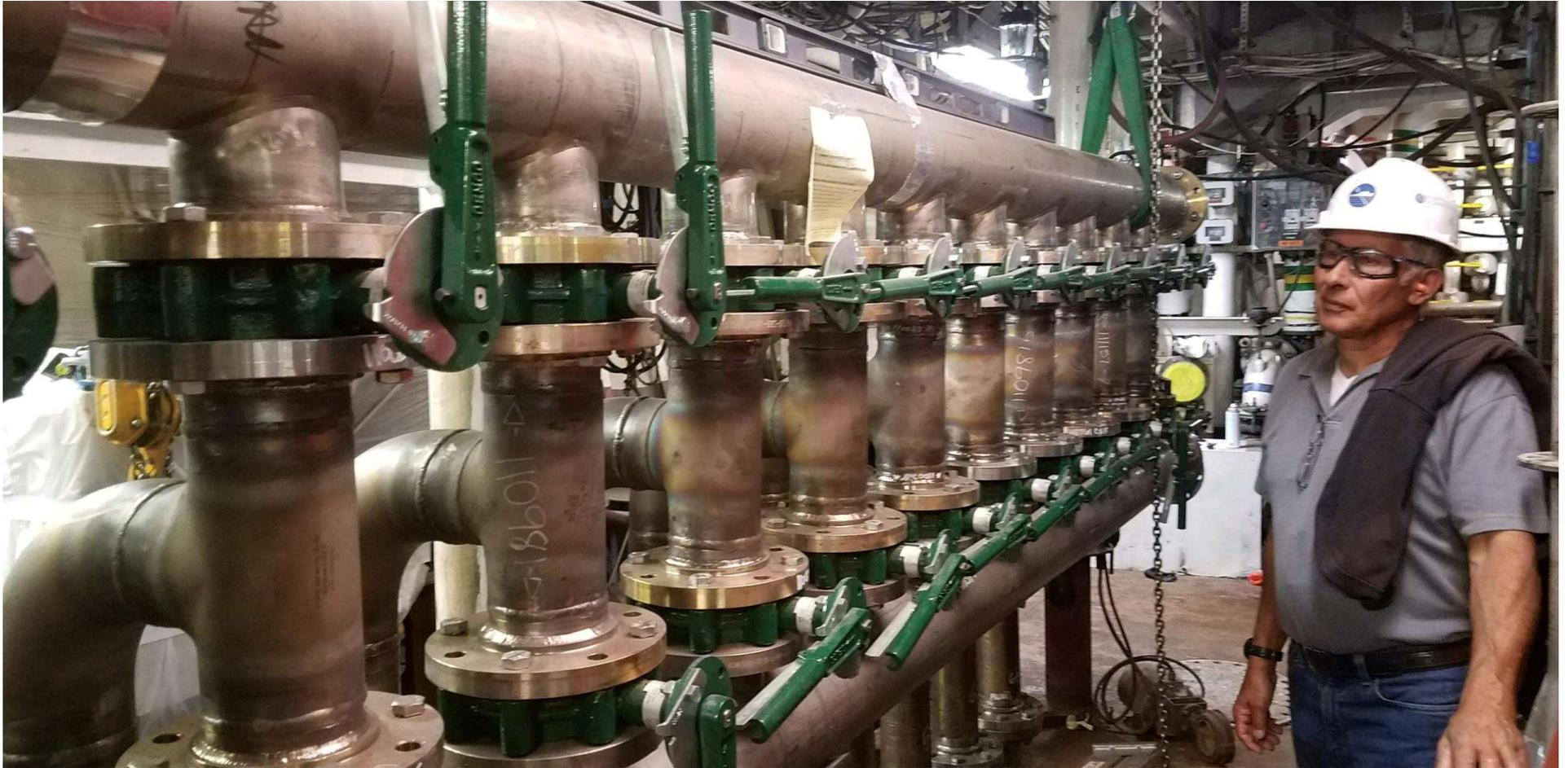
USCG type-approved Optimarin Ballast Water Treatment System along with all new Ballast Water Piping and Manifold
