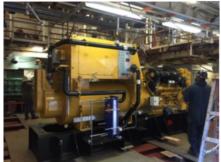
First New Generator moving in
