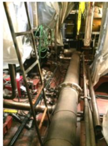
New piping systems
