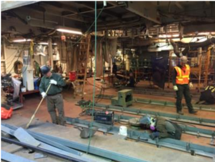
Empty Engine room
