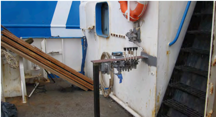
Relocated crane controls
