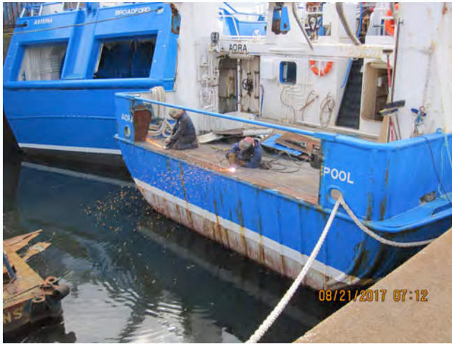
Stern Bulwark Removed
