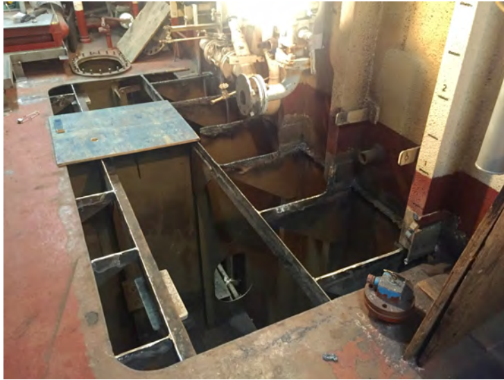
Sewage Tank Top Plating Repair
