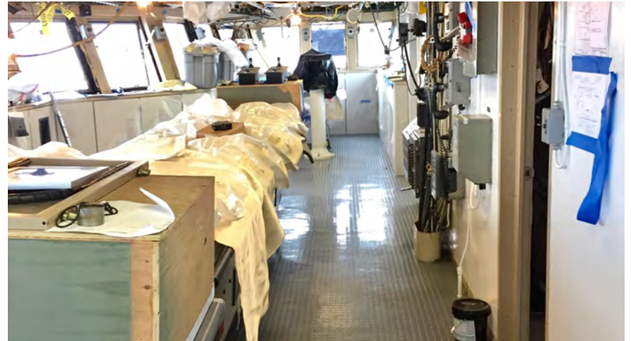
Pilothouse coming together
