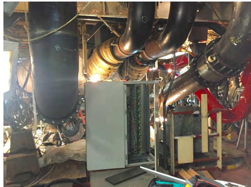
UNOLS Fall 2017 Diesel exhausts entering the stack 6
