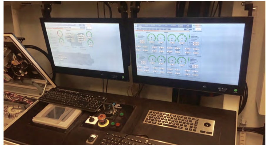
Engineer's Operating Station at initial lite-off
