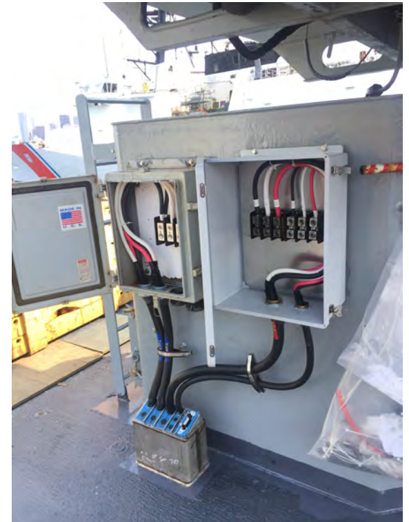
New 400 Amp Aft Deck Science Power
