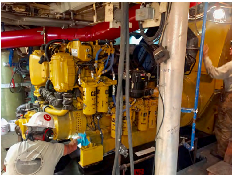
9/8/17 #1 C32 diesel lite-off
