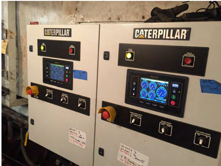
3516 diesel local controls powered up
