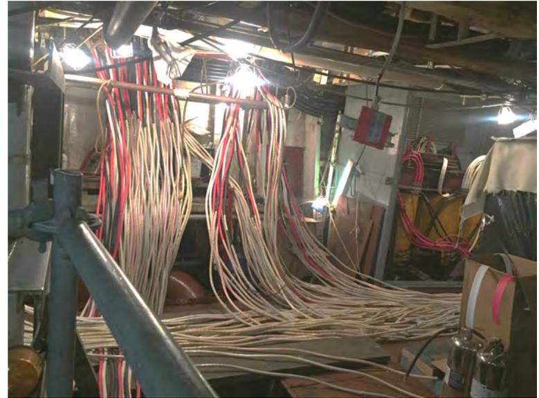
Cables prepared for feeding into switchboards
