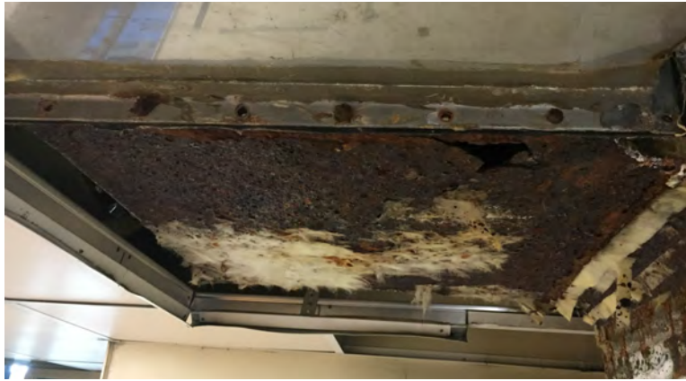
Badly corroded vent ducting
