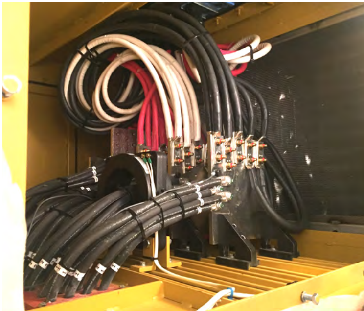
Cable connections in new generator
