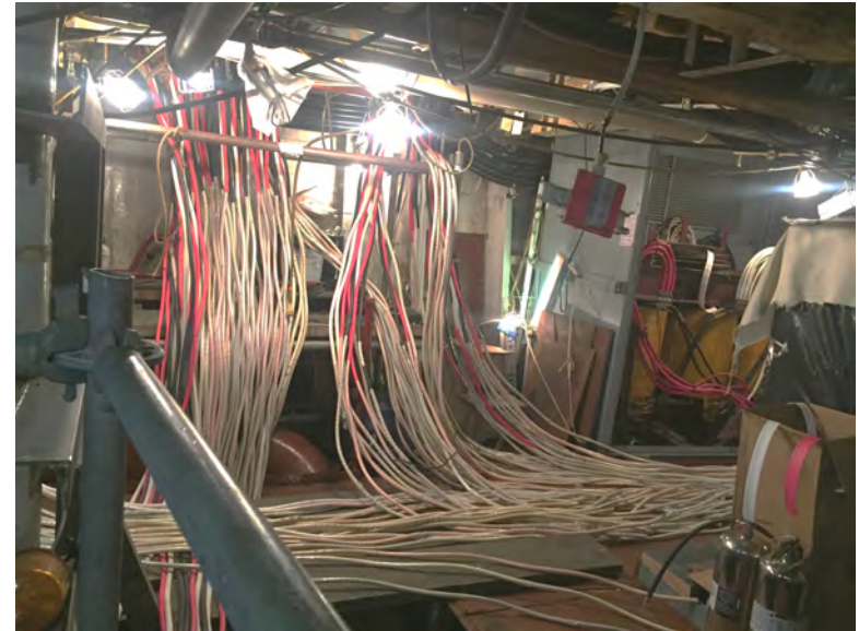
Cables prepared for feeding into switchboards
