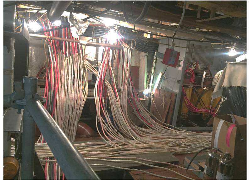
Cables prepared for feeding into switchboards
