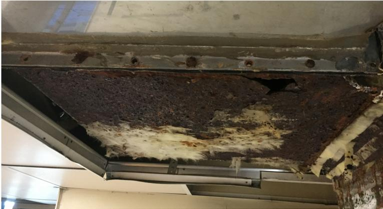
Badly corroded vent ducting
