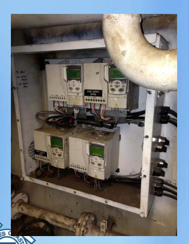
Example: Cruise Ship experienced motor controller overheating and eventual failure.
