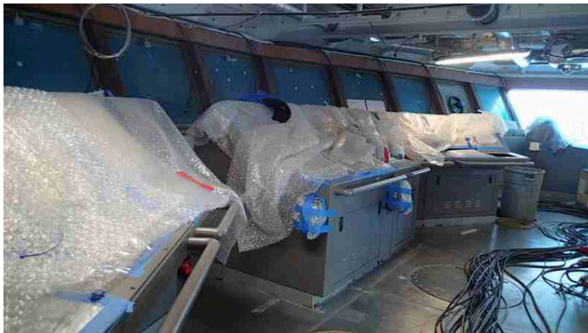
Bridge Consoles being installed
