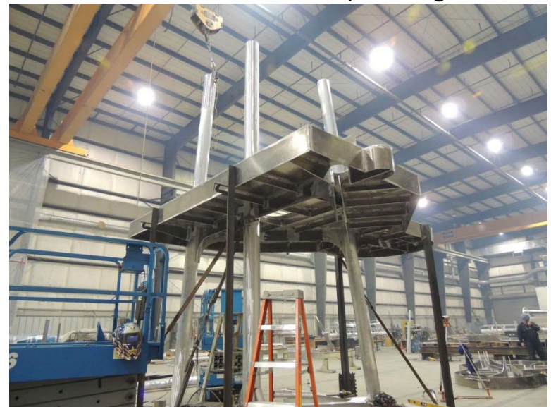
Mast Under Construction
