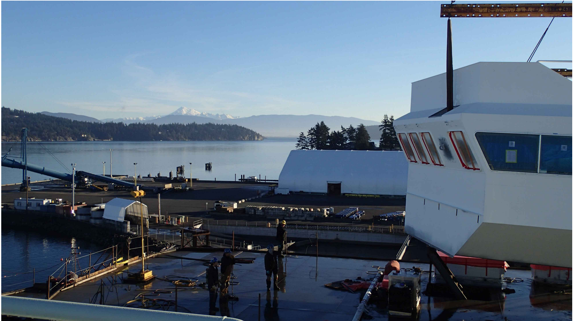
Pilot house being landed on Sally Ride
