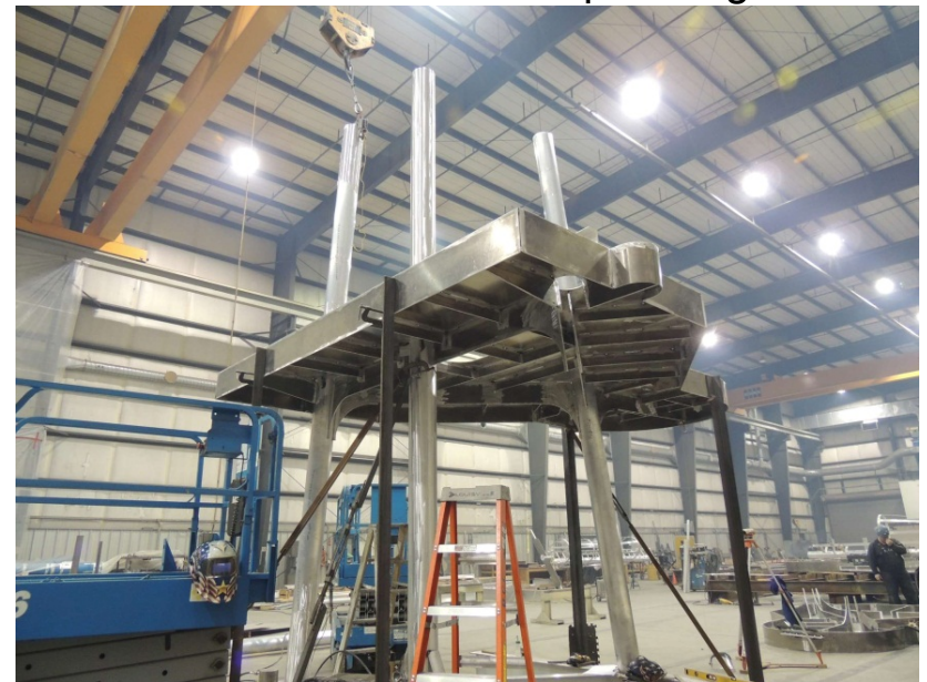
Mast Under Construction
