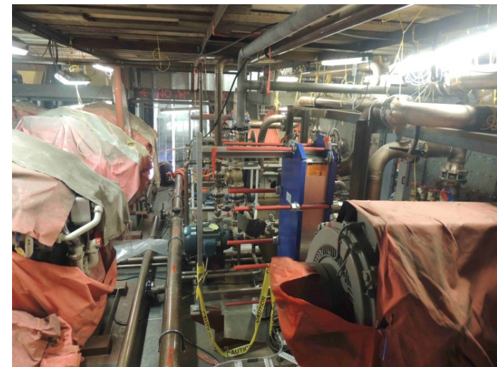
Engine Room filling up with equipment
