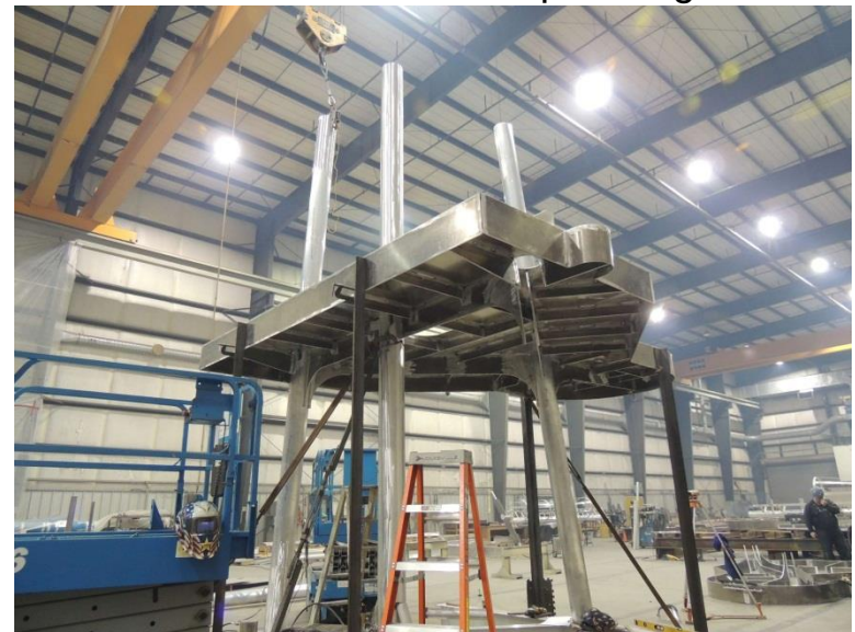
Mast Under Construction
