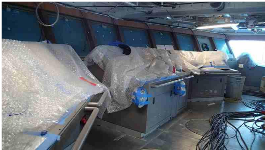
Bridge Consoles being installed
