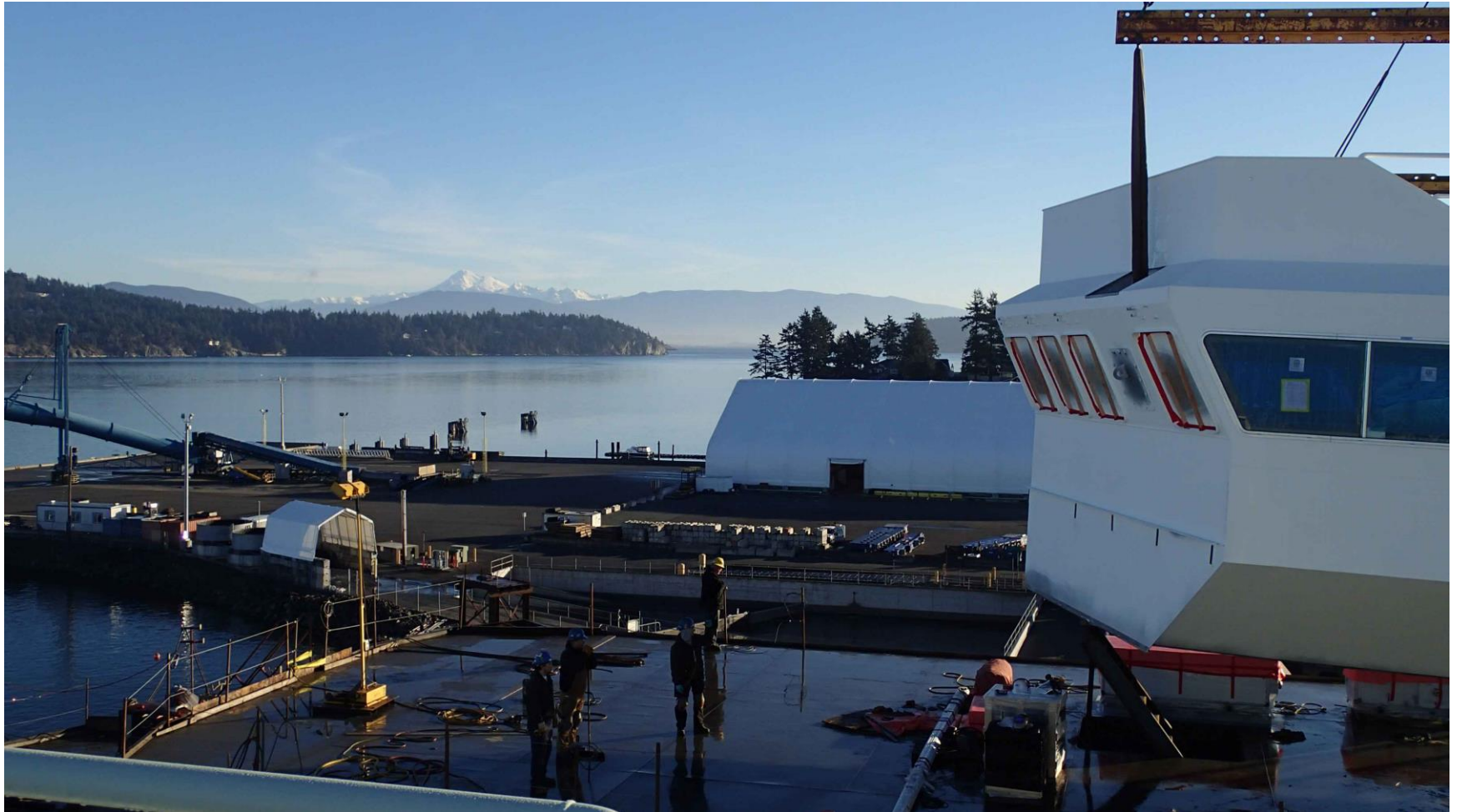
Pilot house being landed on Sally Ride
