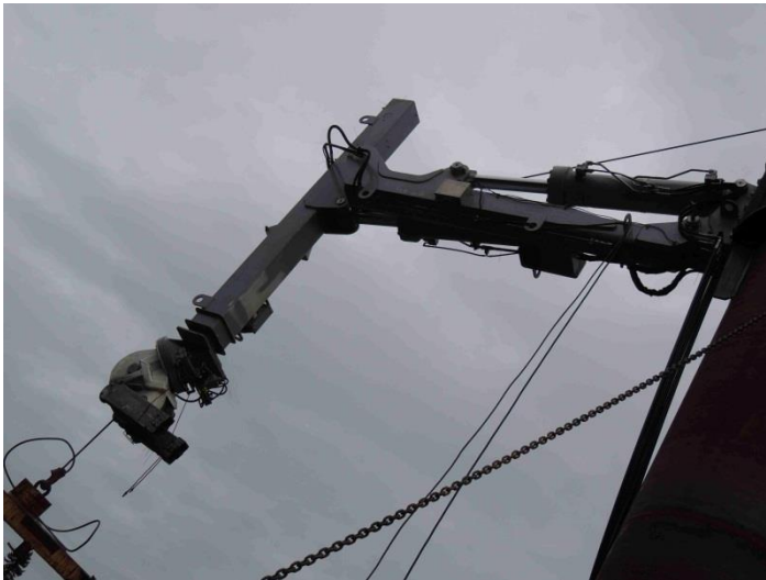
Handling System FAT - Allied
