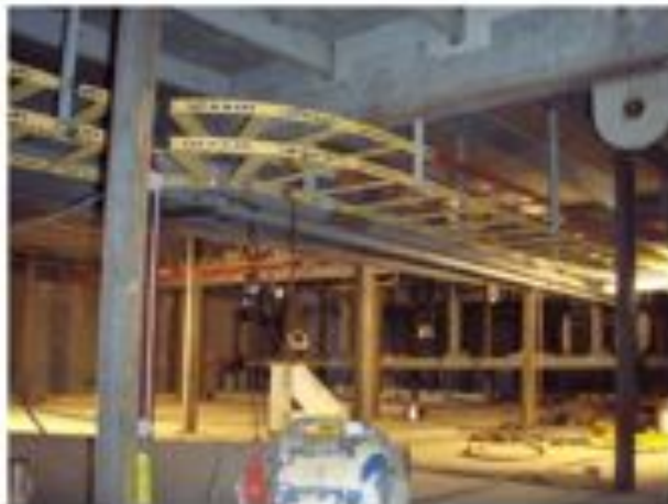
Machy Space Wireways in overhead
