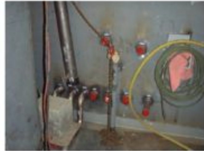
SW bulkhead penetration
