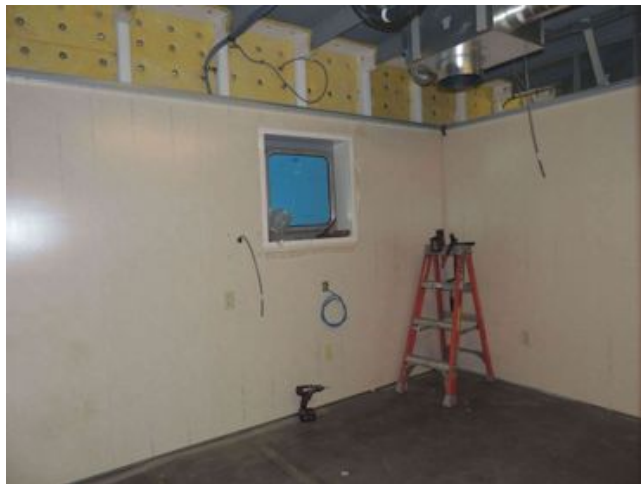
Stateroom joiner work, insulation, port light
