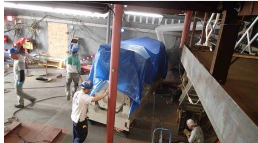
Moving Genset into place
