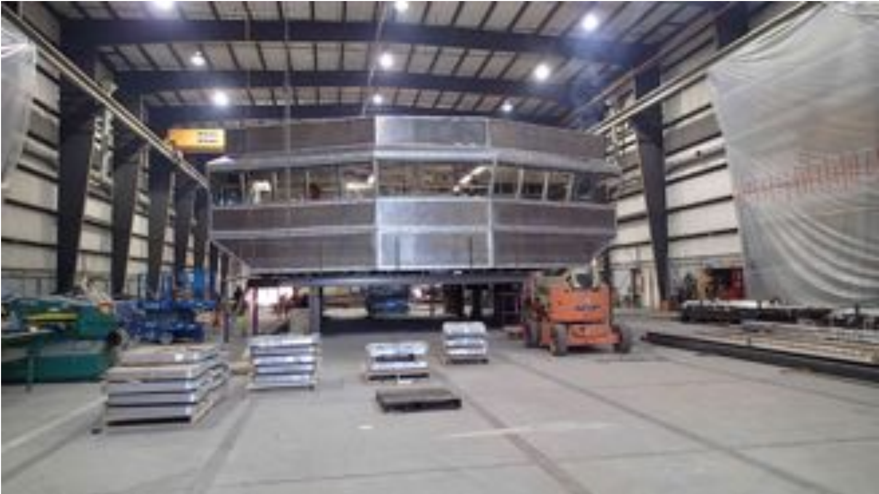
SALLY RIDE Pilot House nearing completion in the “Big House”
