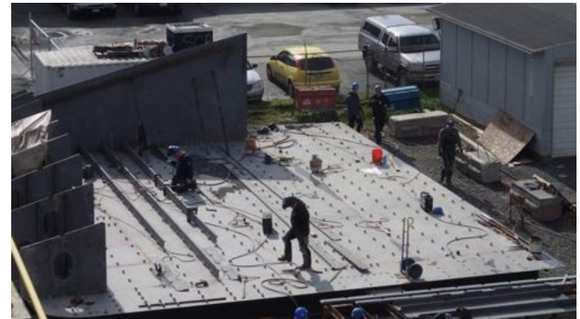
AGOR 28 Main Deck – Upside Down – Bolt Holes
