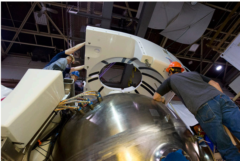
Installing top-forward section of foam
