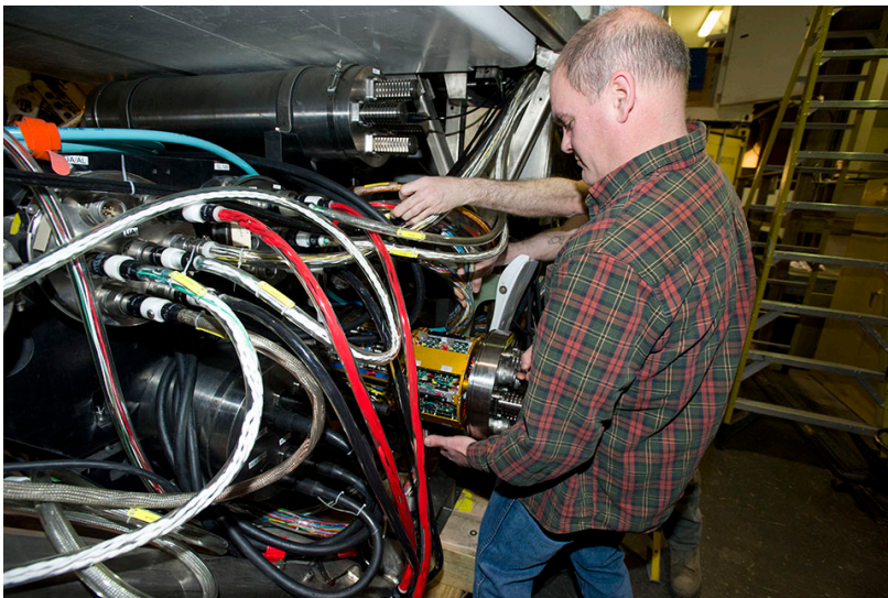
Installing power distribution controller
