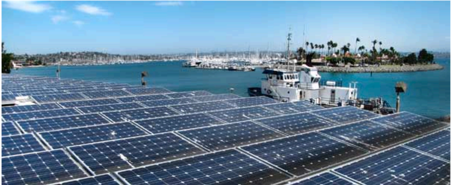
Nimitz Marine Facility installs photovoltaic system
