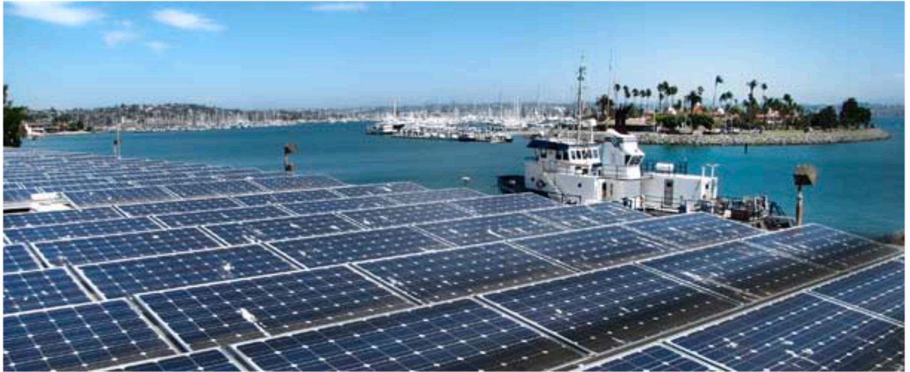
Nimitz Marine Facility installs photovoltaic system
