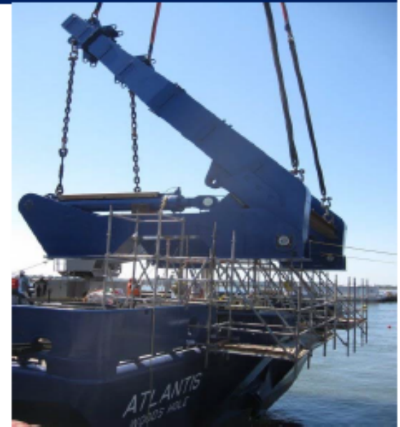
Installing the A-frame March 2011
