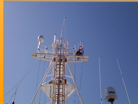
Antenna placement and cable run
