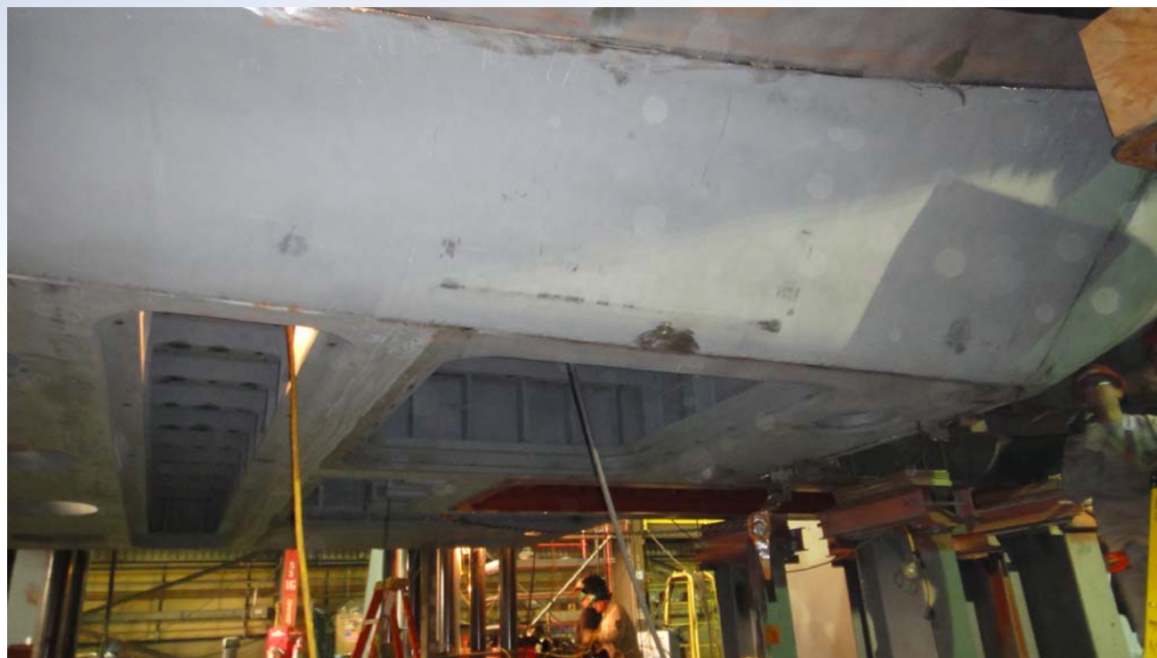
ARRV (0650) MV SIKULIAQ PROGRESS PHOTO DATE: 10-14-11 CONTRACT NO.: UAF-10-0040 DESCRIPTION: Transducer Flat
