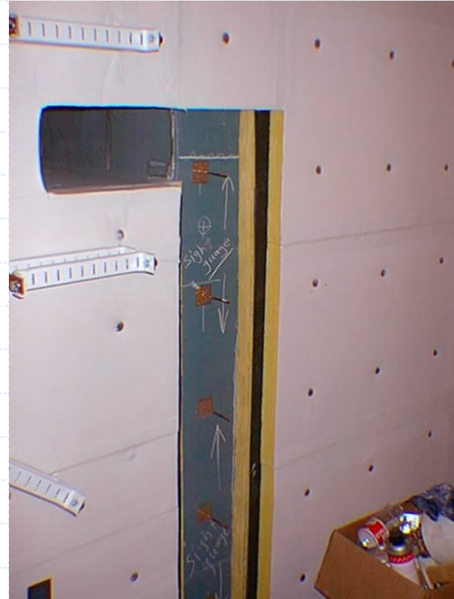
Opening in Insulation during Construction.
