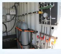
Plumbing for up to 4 storage bank tanks with all fittings and tubing rated to 5000 PSI.
