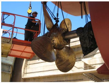
Shipyard forced to remove prop and shaft to remove tallow over Christmas break AND pay consequential damages for loss of charter hire
