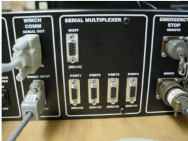
Lab Deck Box – Rear showing some of the connections to deck cable.
