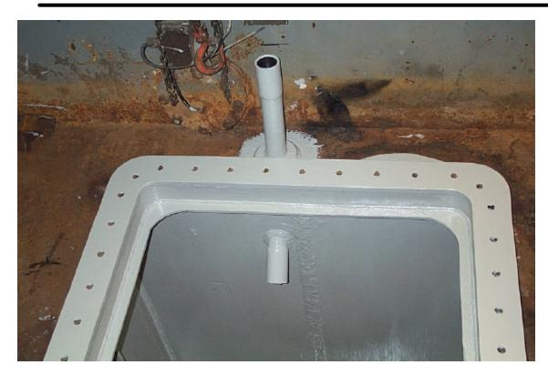
Conduit extends above waterline Rox-tec glands installed at top and bottom
