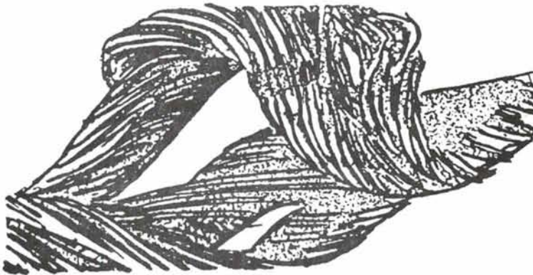
Birdcage which has been forced through a tight sheave
