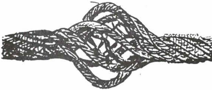
Birdcage caused by sudden release of tension and resultant rebound from overloaded condition
