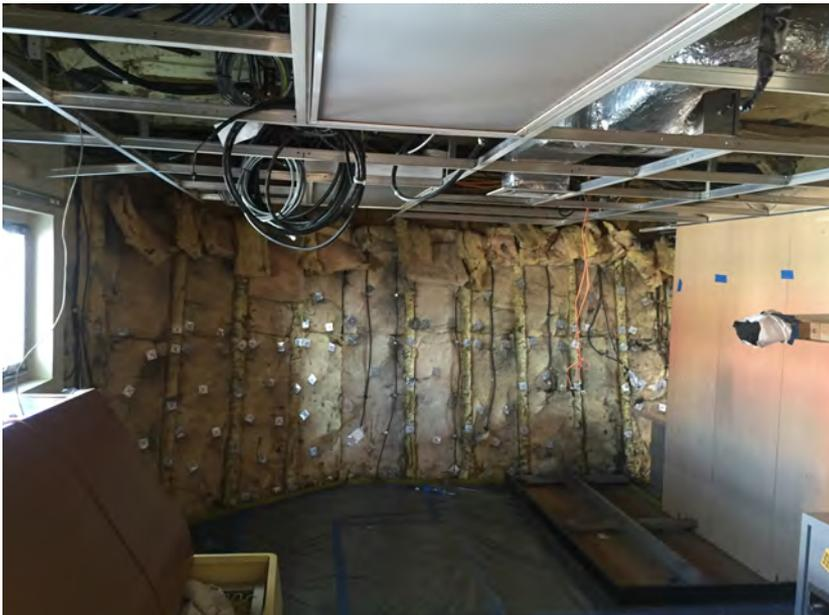
Installation of new catwalk forward of the space, new cable feeds to new Bridge consoles above
