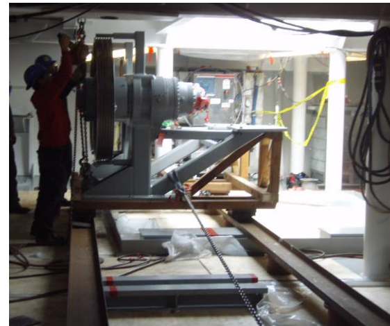
Markey Traction Winch being installed
