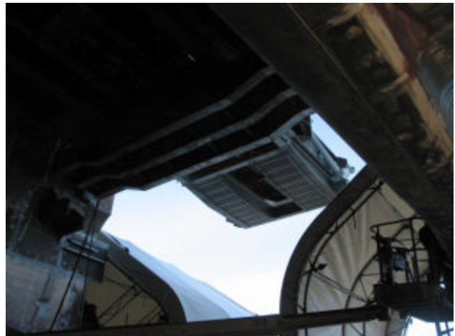
Stern Ramp from below
