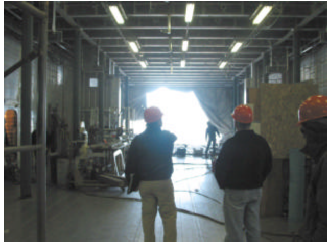
Interior View – looking aft
