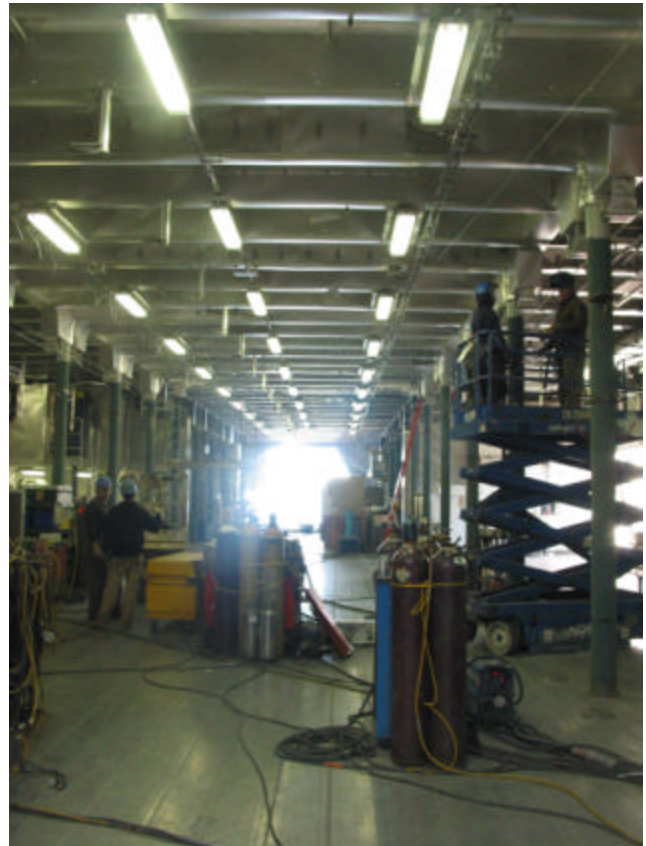
Long View Aft
