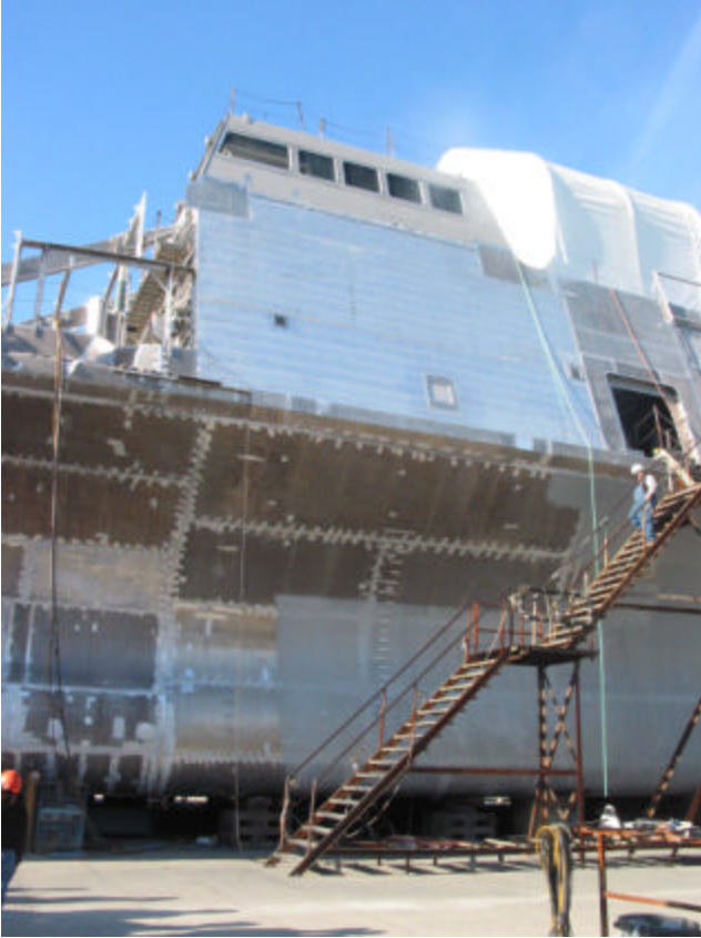
Port side Metal Fabrication
