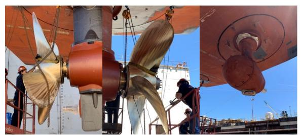
Propeller being installed on Starboard Z-Drive
