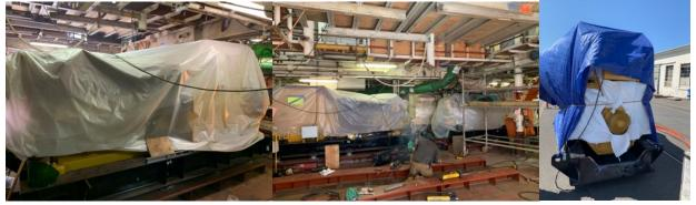
C32 installed and foundation for first 3516 being welded in place; 3515 with modified skid
