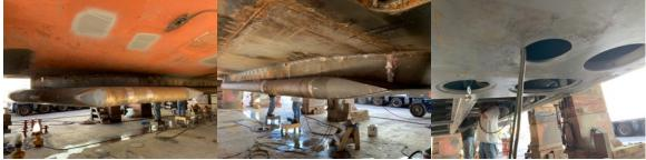
Gondola installed and welled to hull and being prepared for painting
