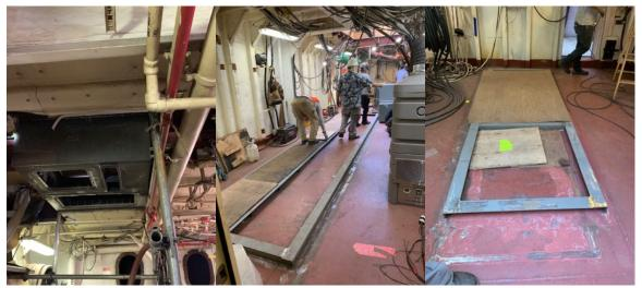
Riser boxes and foundations almost ready for installation of switchboards
