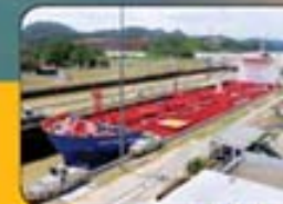
> The current draft in the existing locks is 108'. Post-Panamax vessels 160' wide will pass through the new channel.
