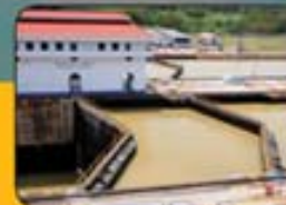
> The existing locks structure displaces a great deal of water from Gatun Lake. The new design will use 7% less water.
