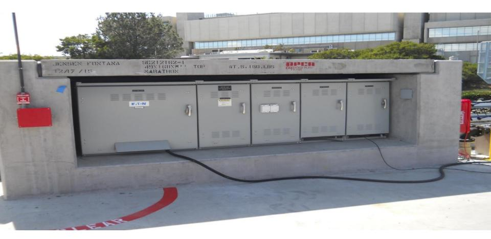
All ship's loads including crane and winch starting current can be picked up on shore power
