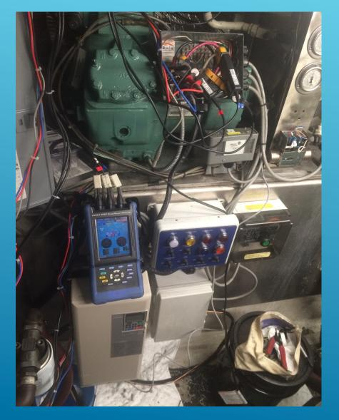
VFD: Most efficient way to control compressor capacity
