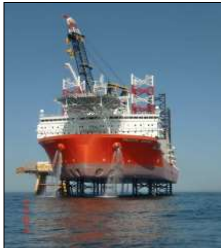
Mechanical Equipment Subject to Immersion
