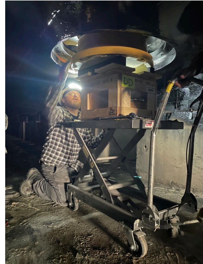
EK80 Transducer Installation
