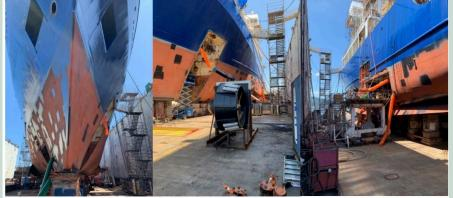
Hull with openings for thruster and engine install, one coat of A/C paint
