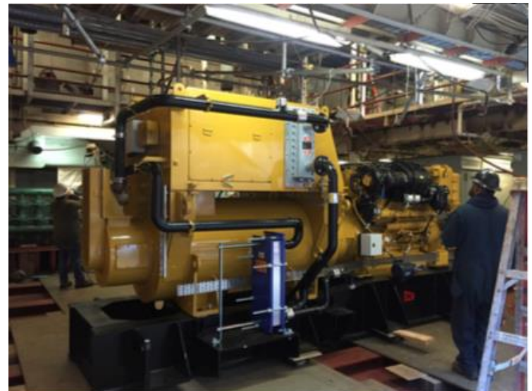
First New Generator moving in
