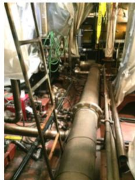
New piping systems
