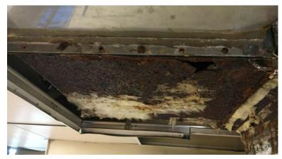
Badly corroded vent ducting
