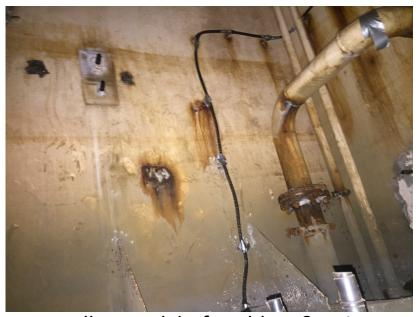
Ballast tank before blast & paint
