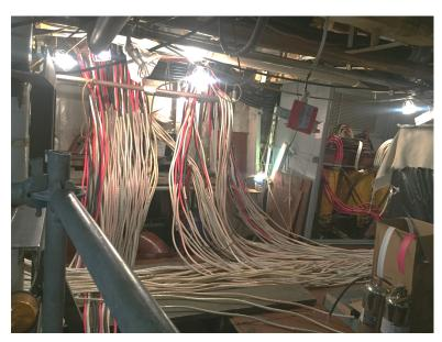
Cables prepared for feeding into switchboards
