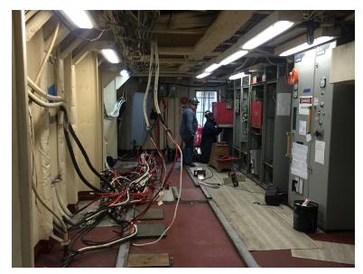
Old Switchboards & Drives being removed
