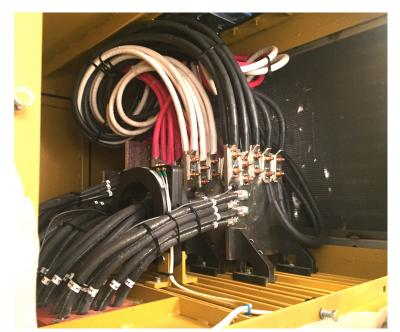
Cable connections in new generator
