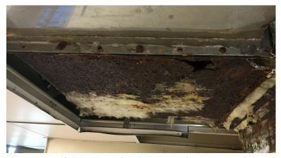
Badly corroded vent ducting
