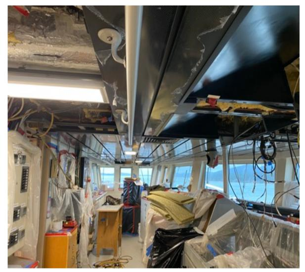
KONGSBERG DP SYS UPGRADE **NEW VHFs** NEW WHISTLE CONTROLLER NEW GYRO REPEATERS **NEW WIND BIRDS – ULTRASONIC NEW ZDRIVE CONTROLS** SIEMENS SYSTEMS DISPLAYS NAV LIGHTS UPGRADES – LED **GMDSS UPGRADES FCDIS REMAINING** PA SYSTEM RENEWAL FULL RESKINNING OF ALL CONSOLES AND FIDDLEBOARDS **NEW OVERHEADS AND LIGHTING NEW DECKING**
