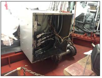
Propulsion motors to remove, disassemble, clean, inspect & test
