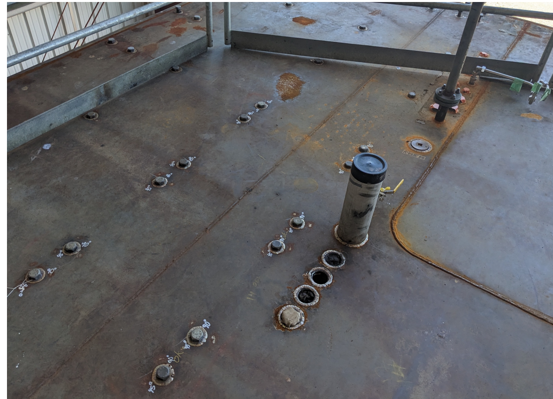
Deck socket testing V2
