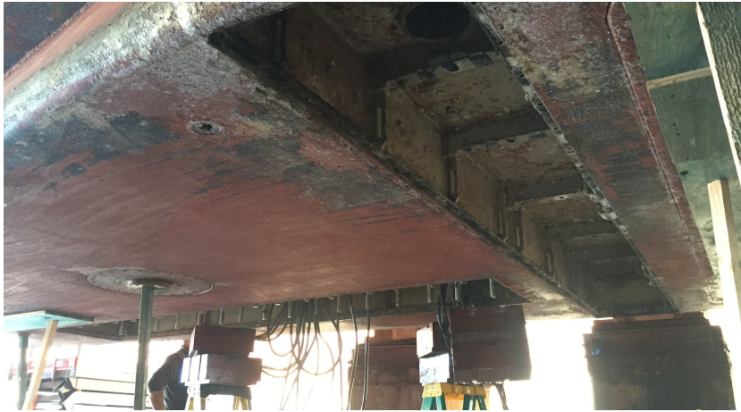
EM-302 being replaced
