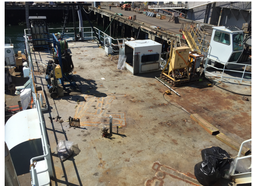
Heavily corroded O2 Deck
