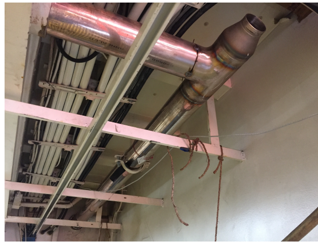
New firemain piping
