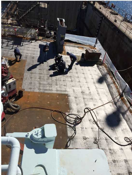
4/16/17 Blasting the aft main deck
