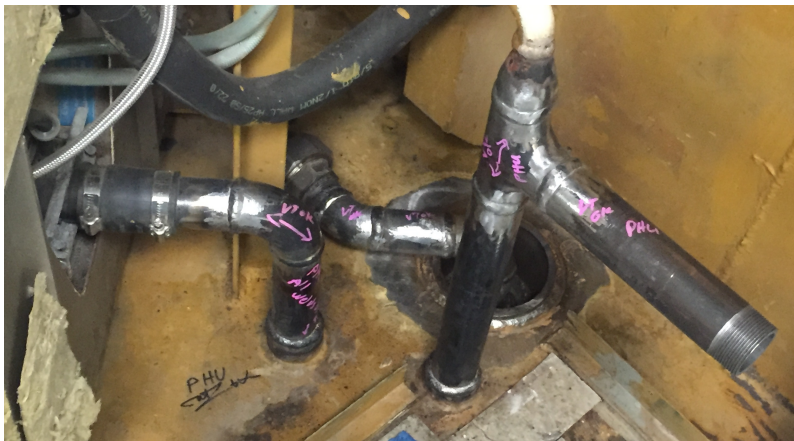
New drainage piping for head modules
