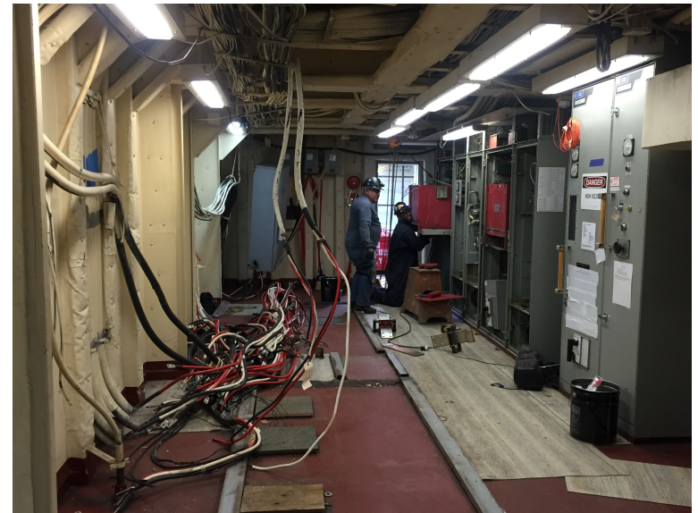
Old Switchboards & Drives being removed
