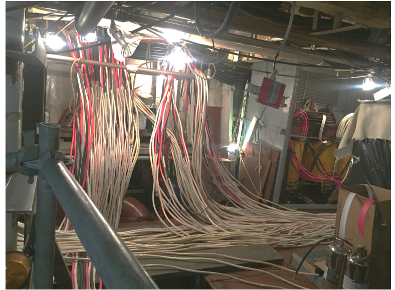
Cables prepared for feeding into switchboards
