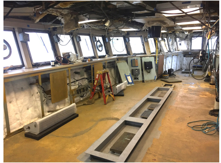
Bridge gutted & prepped for new consoles
