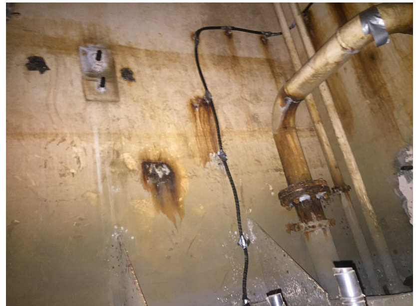
Ballast tank before blast & paint
