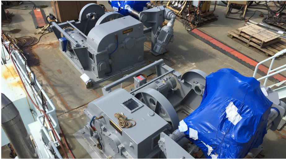
Refurbished hydro-winches in place
