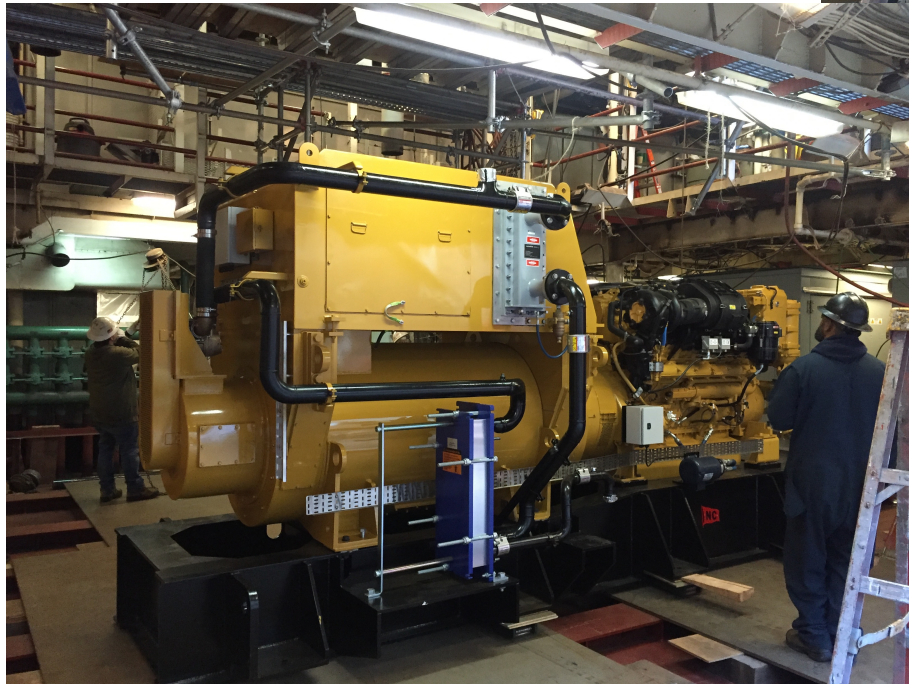
First new generator set being moved into place
