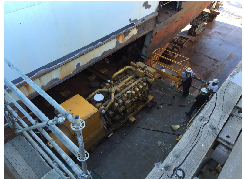
1 st generator set out
