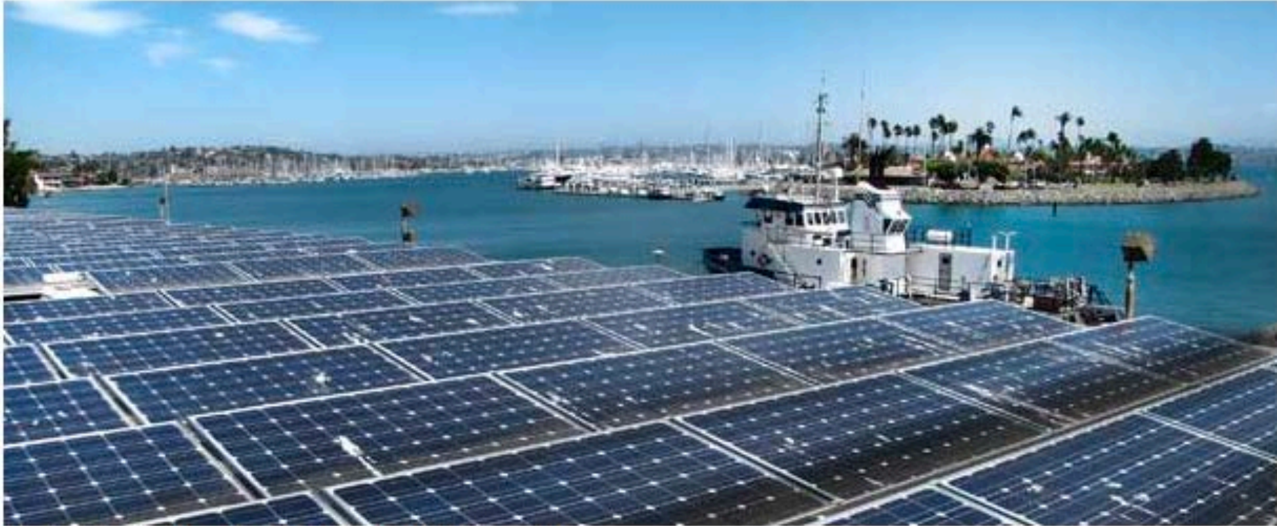
Nimitz Marine Facility installs photovoltaic system
