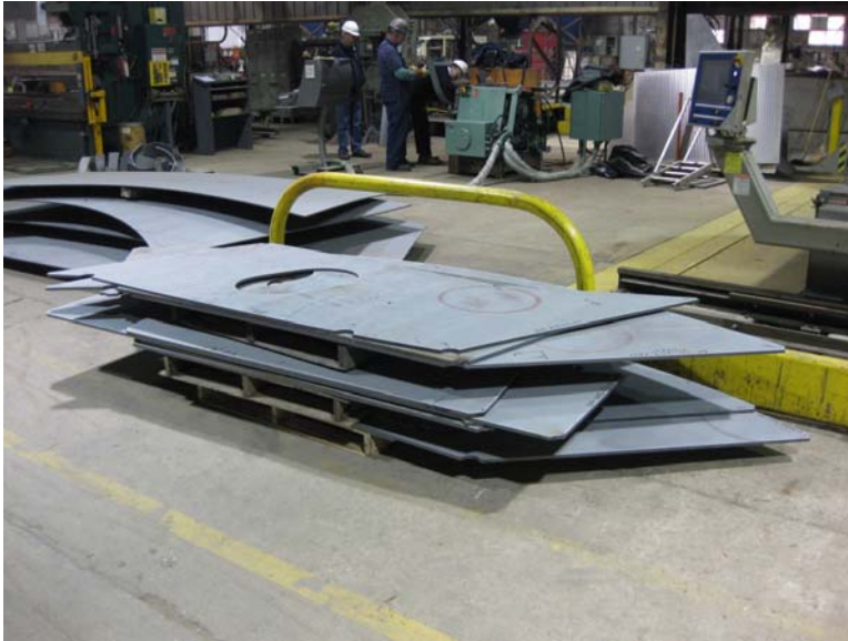
Figure 3: After being cut, the various pieces are staged for assembly into panels.
