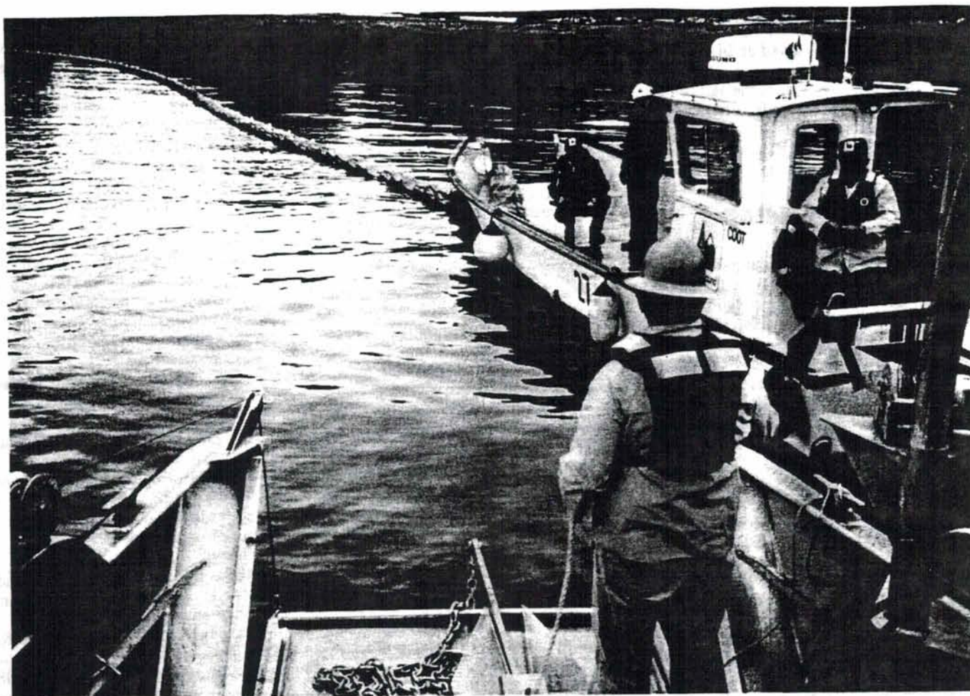
Fast-Response boats deploy boom through an open ramp at the bow.
